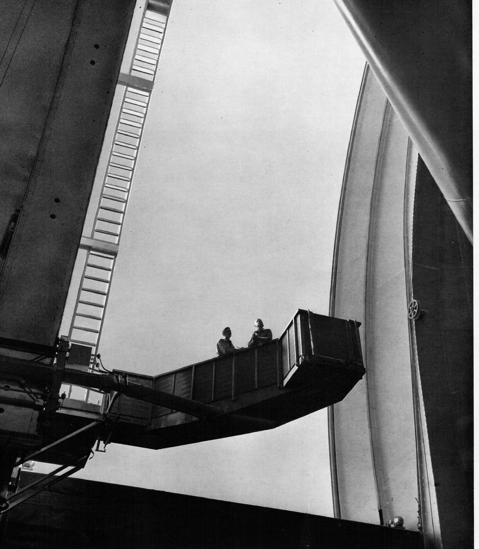
The two men in the picture are riding the elevator in the 200-inch telescope dome, with the opening slot of the dome behind them. This elevator carries the astronomer up to a point where, with the telescope tube tilted into proper position, he can step across into the observer's "cage," which is at the prime focus in the upper end of the tube. The picture on page 32 shows an astronomer at work in the cage.
